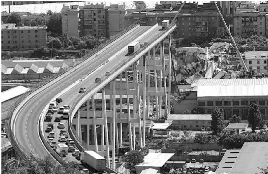
Figure 4.2 The remains of Morandi Bridge, after a section of the bridge collapsed
